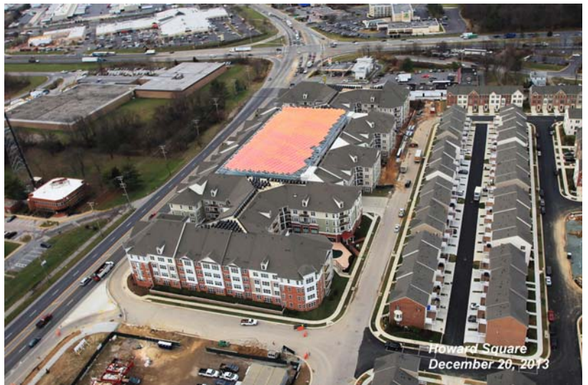
AERIAL PICTURE OF SOLAR ARRAY
